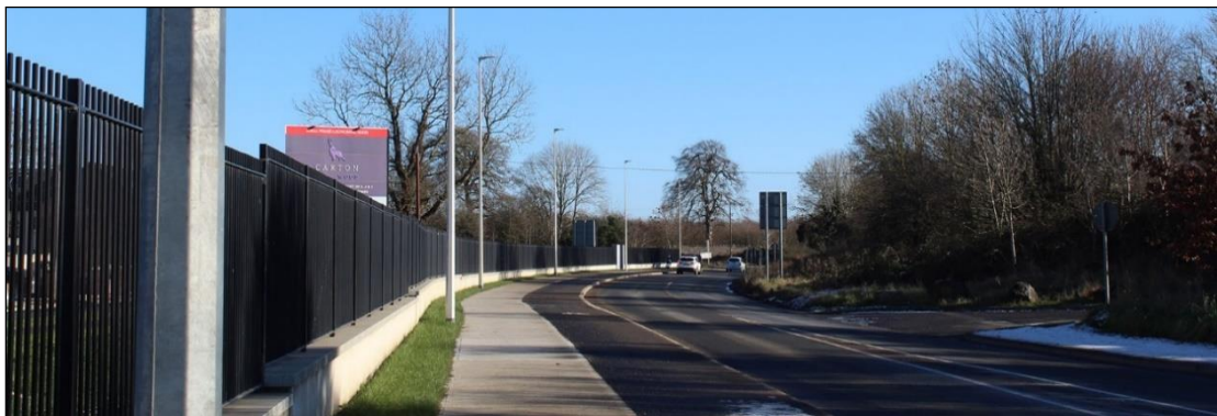
Figure 4.23 Carton Wood housing development northwest of R148/R157 junction
