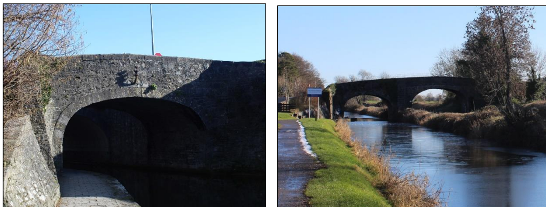
Figures 4.27 & 4.28 Mullen Bridge from the west, and Pike Bridge
